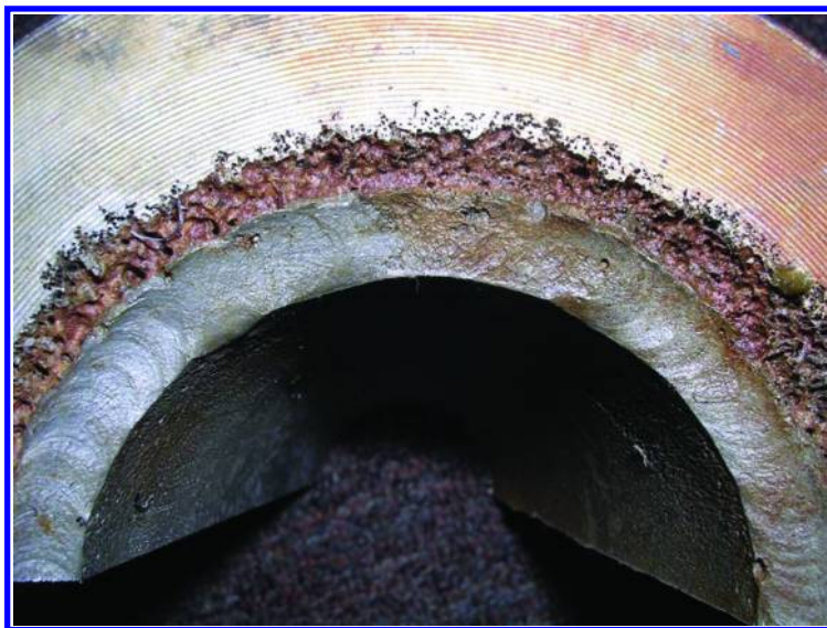
Figure 3. Heat affected zone of weld at discharge flange (Hastelloy). (see color insert)
